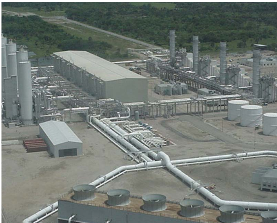
The four nitrogen-production units stand at the right in the view of the Cantarell nitrogen-generation plant. Photograph from Compañía de Nitrógeno de Cantarell and Petróleos Mexicanos.
